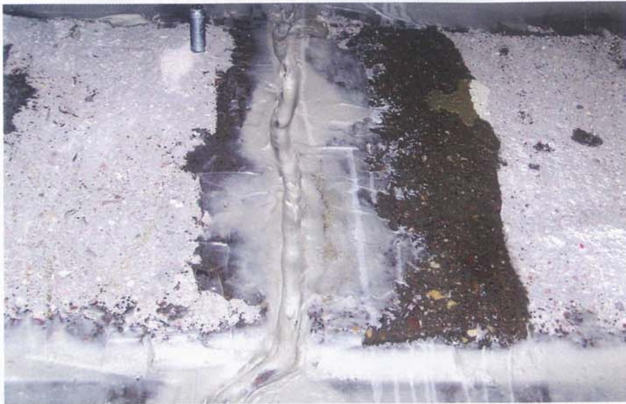
View of the ICO-Gel product being applied to Upper Stillwater Dam
