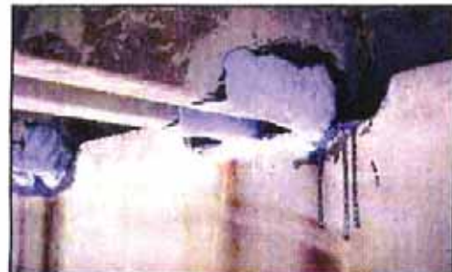
Workers applied patch material to areas of severe wear on bridge girders (above). In areas of severe flexing, braces held material while patch set (below).
