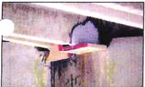
Workers applied patch material to areas of severe wear on bridge girders (above). In areas of severe flexing, braces held material while patch set (below).
