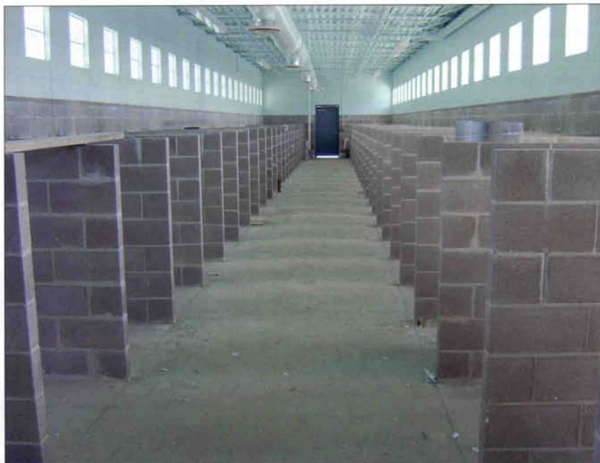
Stone Mountain Pet Lodge is not your average kennel; it's an upscale facility with a 9,000 square-foot kennel area that can board 200 dogs and 75 cats.
