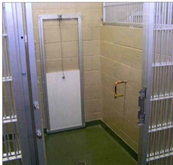
Dogs have their own 4- by 6-foot indoor kennels attached to 4- by 12-foot outdoor kennels. The system used at Stone Mountain Pet Lodge was ICO Glaze epoxy coating system on the block walls, ICO Quartz 120 DB epoxy system on the floors and ICO Quartz Cove providing a seamless transition between the wall and floor.
