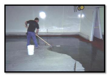
**6000 FS** was installed at ¼" (6mm) over entire processing, cooler and freezer areas to form a monolithic surface with a non-slip surface. The 6,000 ft.² (600 m²) project was completed in 3 days. The vinyl ester floor system has prevented any chemical attack for the four years of service. The **6000 FS** has also withstood the abuse normally experienced from heavy forklift traffic.
