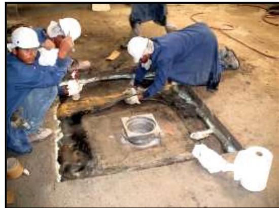
Turning their attention to the floor, Tom and his crew used pneumatic chipping tools to remove layers (some of which were 3-4" in thickness) of previous polymer and cementitious fillers that were poorly bonded to the substrate. The floor was totally disinfected, pressure washed, then acid etched and scarified where necessary to obtain a clean, sound, abraded substrate. In addition, all open cracks were V-notched out and keyways were cut around all drain plates and entryways.
