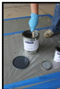
C.) For enhanced safety, an optional, nonskid additive is provided in the kit. This material should be added to the mixed resins in the final coat to reduce the risk of slipping on finished floors that may be exposed to wet conditions. Slowly pour these contents into the mixed resins and stir to suspend throughout the material.
