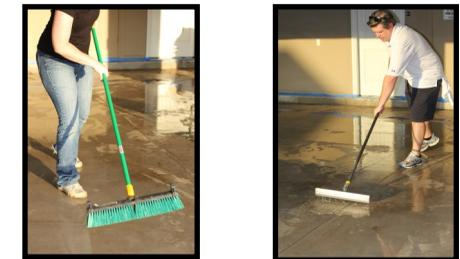
Begin installation when the concrete surface is clean and dry to the touch.
