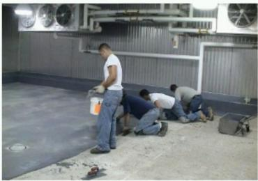
The crew also coated the room's concrete curbs with the ICO Guard 51. "We then caulked the curbs with International Coatings' ICO Lastic Gun Grade to protect against moisture penetration between the concrete and the new stainless steel panels," describes Behunin. ICO Lastic Gun Grade is a two-part, 100% solids, epoxymodified urethane designed as a moisture barrier for use in interior situations where moderate movement is expected—such as expansion joints.
