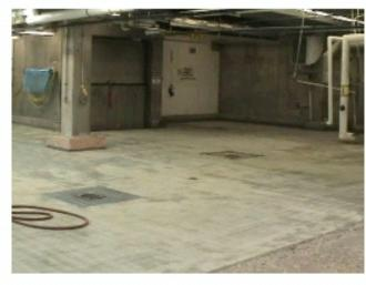
collapse into the holes." They also cut and filled keyways around all drain plates and at the entryway to the room. When the epoxy had cured, the floor was washed with hot water.
