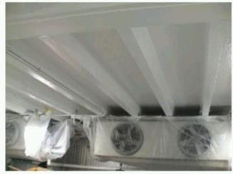
0.36mm) each, backrolling to ensure coverage. This was followed by one, 10 to 15 wet mil (0.25mm-0.38mm) top coat of ICO Glaze Top Coat." The ICO Glaze Top Coat is a high gloss, 100% solids, epoxy that is designed to provide a complete vapor barrier able to withstand the cooling room's constant damp and sanitizing chemicals.
