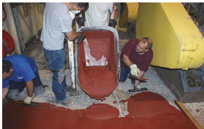
ABOVE ▲ "To create the slope," Behunin says, "we had to build the floor up to a thickness of 3" (7.62cm) in some places, tapering down to ¼" (0.64cm) at the drain."
