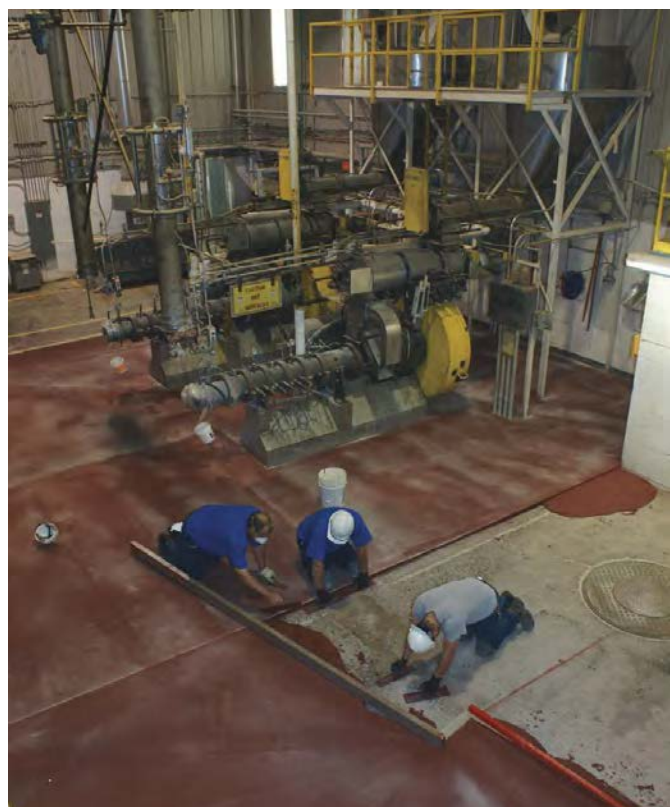
ABOVE ▲ "To create the slope," Behunin says, "we had to build the floor up to a thickness of 3" (7.62cm) in some places, tapering down to ¼" (0.64cm) at the drain."
