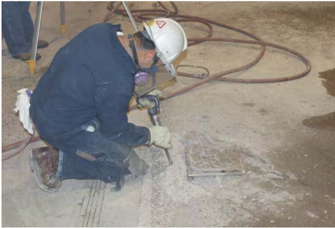
ABOVE ▲ The Behunin crew used Ingersoll Rand air saws, pneumatic chipping hammers, and scaling hammers to remove delaminated coating and unsound concrete.
