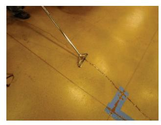
epoxy repair materials. "The process of filling a joint is relatively simple," he explains. "First, the crack needs to be chased using a saw. Then the semi rigid polyuria is applied to the crack; this is usually done using a two-part cartridge that automatically mixes the two substances." Christensen stresses the importance of making sure the crack is slightly overfilled. After the material has been applied, it must be given a brief period of time to dry. Once this is done, the
