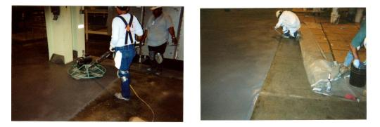
To provide a good profile the floor was shot blasted. All cracks and deteriorated areas were repaired. A key was cut around all drains and the entire periphery. The floor was primed with ICO Primer LV Fast Cure to minimize the curing period required before placement of the ICO Guard 51. At 60°F - 65°F the primer cured in 2 hours, (approximately the same time required to coat the 4,500 sq ft).
