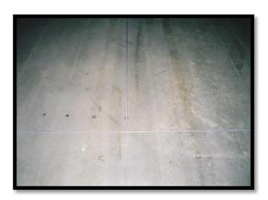
The 1000 CS has shown excellent durability for the 5 years of service. Tow motors and forklifts have produced minimal wear in the aisle ways.
