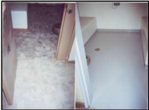
The floors have added difficulty as they are subjected to harsh cleaning, constant traffic and must be skid resistant. The best performing material found by institutions for this area is the ICO Floor Coating also seen in the finished photo. The system includes ICO Primer LV, and two coats of the Floor Coating. The first coat receives a broadcast of aggregate to provide the required skid resistance needed in shower areas.
