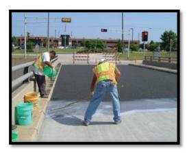
After the second coat was hard enough for foot traffic, the crew swept up all the loose aggregate. The bridge was then opened to traffic, less than 11 hours after the project was started. The project started in the morning by abrading the surface so the coasting system would bond. A worker applied the first coat of epoxy with a squeegee at a rate of 30 square feet per gallon. The
