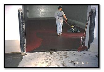
The sealed finished of the **3300 FS** has eliminated the standing water in the spalled concrete where the potential for bacteria growth existed. Wear from forklift traffic has also been greatly reduced. The **3300 FS** has been in service for 7 years and has required no additional maintenance.
