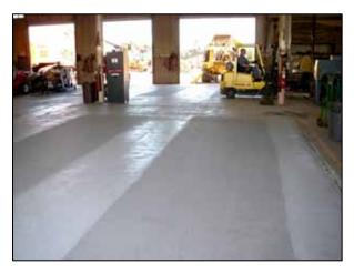
tracked the concrete to obtain a clean, sound, abraded surface for the epoxy to bond with. They also routed out any cracks and pre-filled some of the deeper holes and more severely spalled area.
