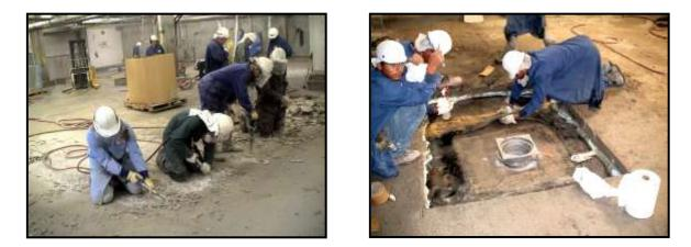
Turning their attention to the floor, Tom and his crew used pneumatic chipping tools to remove layers (some of which were 3-4" in thickness) of previous polymer and cementitious fillers that were poorly bonded to the substrate. The floor was totally disinfected, pressure washed, then acid etched and scarified where necessary to obtain a clean, sound, abraded substrate. In addition, all open cracks were V-notched out and keyways were cut around all drain plates and entryways.
