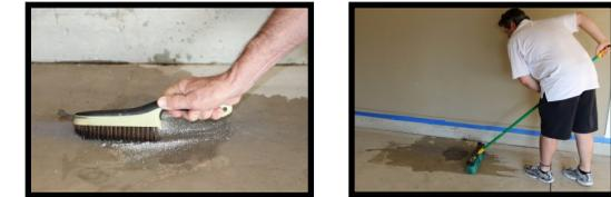
After solution has been allowed to soak for 10-15 minutes, thoroughly rinse the entire surface with plenty of fresh, clean water to remove all Cleaner/Degreaser. Broom and/or squeegee off any puddles of water prior to beginning the installation.
