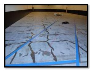
Being located in Tampa Bay, FL, humidity and rain caused American Garage to re-think their strategy for laying down the flooring. Unexpected conditions meant there were no climate controls available leaving the space to be around 85°F inside. The ICO Floor Coating bonded extremely well, but when attempting to use the Ureguard 80 they had to stop because it was setting way too fast due to the temperature and humidity.
