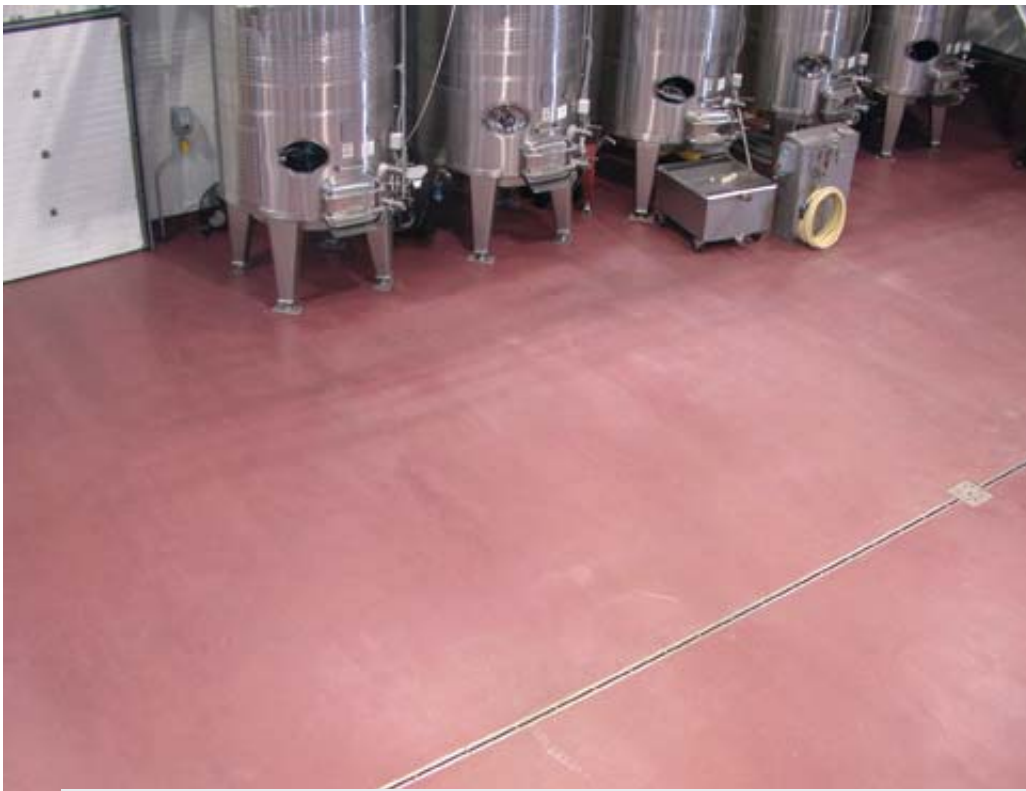
A sanitary work surface drains directly to stainless gutters.
