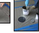
C.) For enhanced safety, an optional, nonskid additive is provided in the kit. This material should be added to the mixed resins in the final coat to reduce the risk of slipping on finished floors that may be exposed to wet conditions. Slowly pour these contents into the mixed resins and stir to suspend throughout the material.
